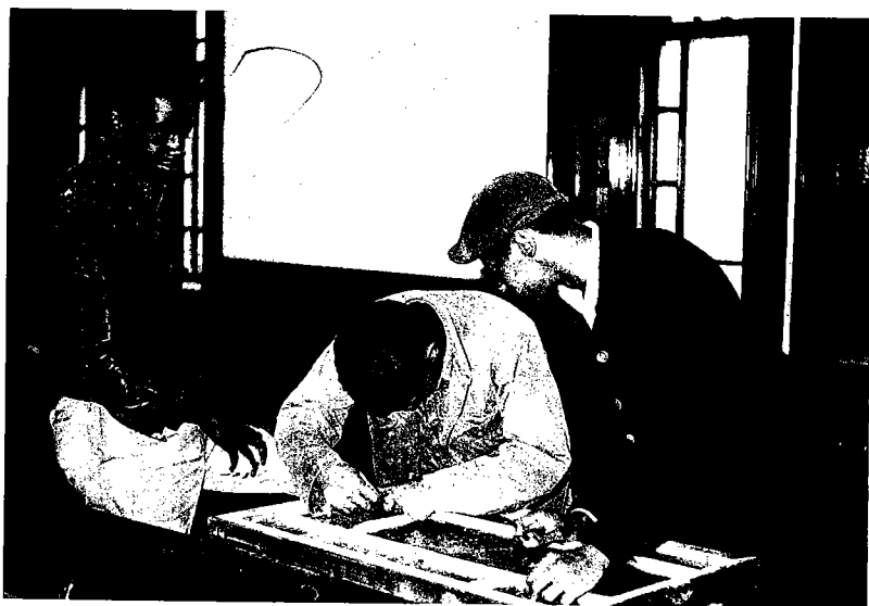
14. A broken window is repaired in Roxbury by trainees in the workcrew project of the youth training and employment program conducted by Action for Boston Community Development (ABCD).
